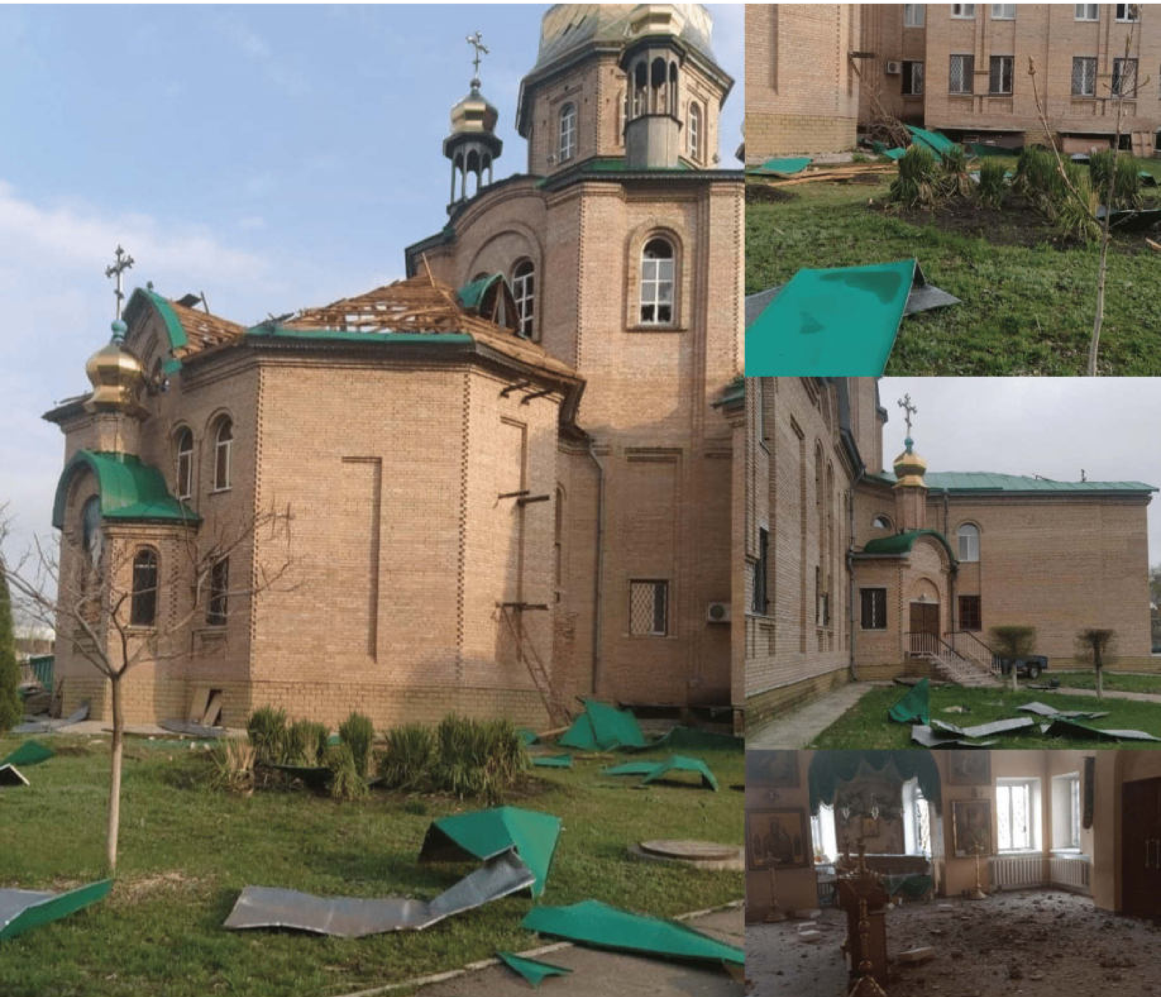
The aftermath of an artillery strike on the building of the cathedral in Severodonetsk (Luhansk region), photo: Serhiy Haidai, 04/17/2022
